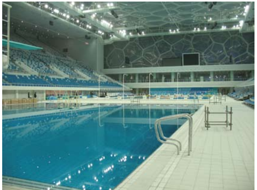
Beijing 2008 Water Cube • Anti Wave Hand Rail
